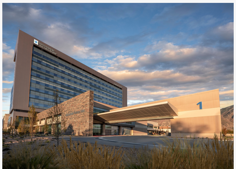
Intermountain Utah Valley Hospital
