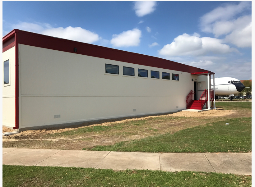
Exterior Side View of the Temporary Modular Office
