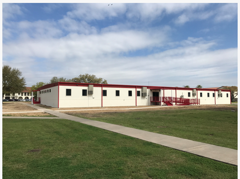
Exterior Front View of the 13,104 SF Temporary Modular Office
