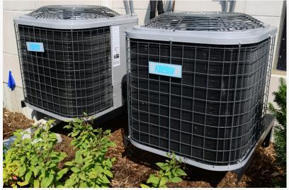
Typically, a central air conditioning unit is composed of an indoor and an outdoor unit. Also, the system consists of air ducts and registers. We will discuss each of the components.
