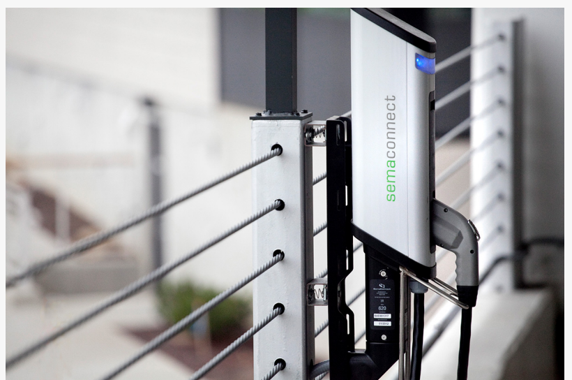
SemaConnect smart EV charging station
