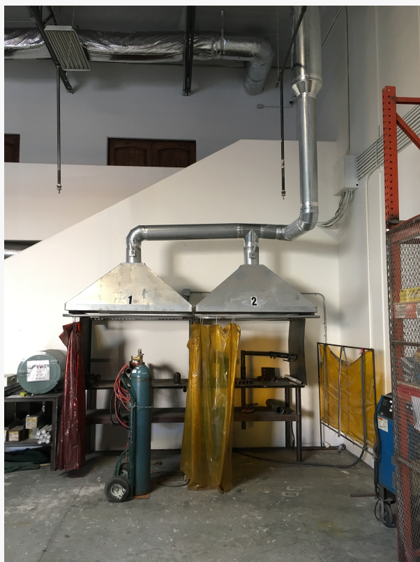
Code Welding and Inspection Shop in Gilbert Arizona
