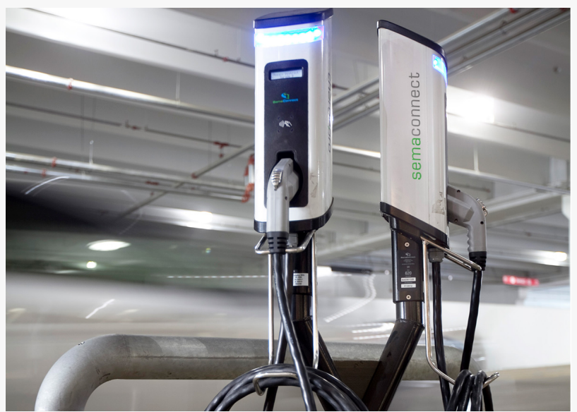
SemaConnect smart EV charging station
