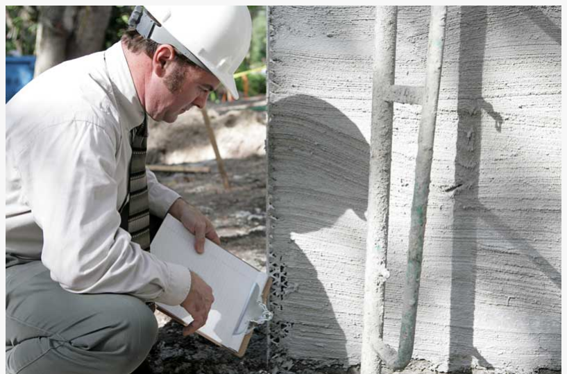
foundation repair contractor inspecting a foundation for damage
