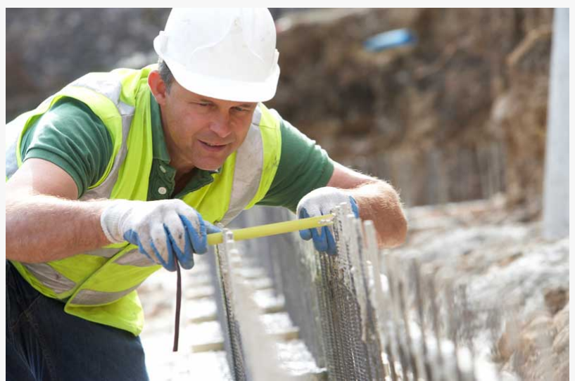
Foundation repair worker measuring a foundation
