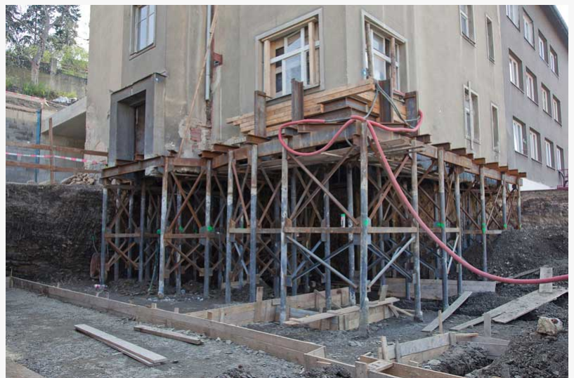
repairing a commercial foundation
