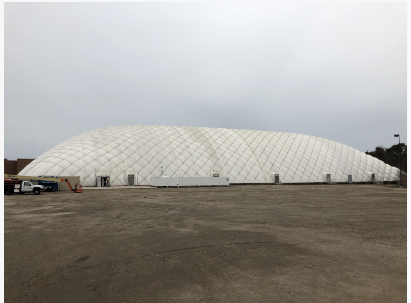
TRRS Bennet Dome Exterior
