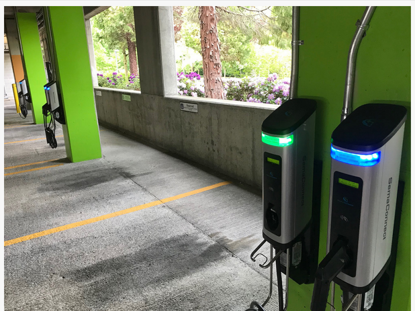
SemaConnect EV charging stations
