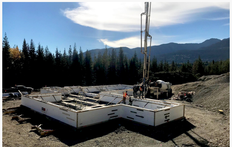
Northern Escape Heli Skiing Lodge under construction
