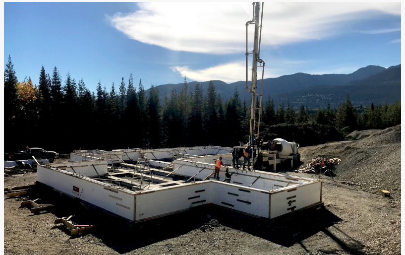
Northern Escape Heli Skiing Lodge under construction
