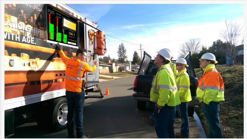
Defects identified and measured in minutes allowing new construction to be certified immediately following installation.
