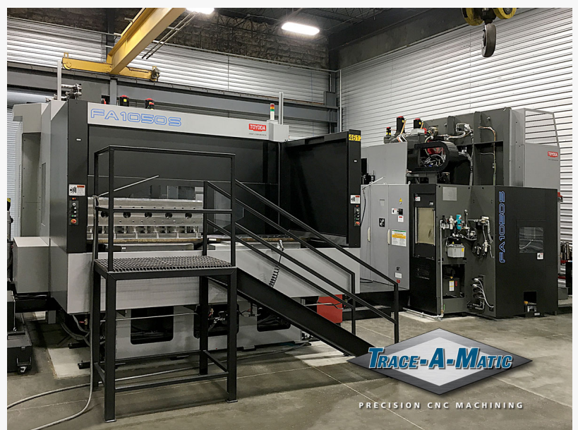
Toyoda FA1050S Installation at Trace-A-Matic South
