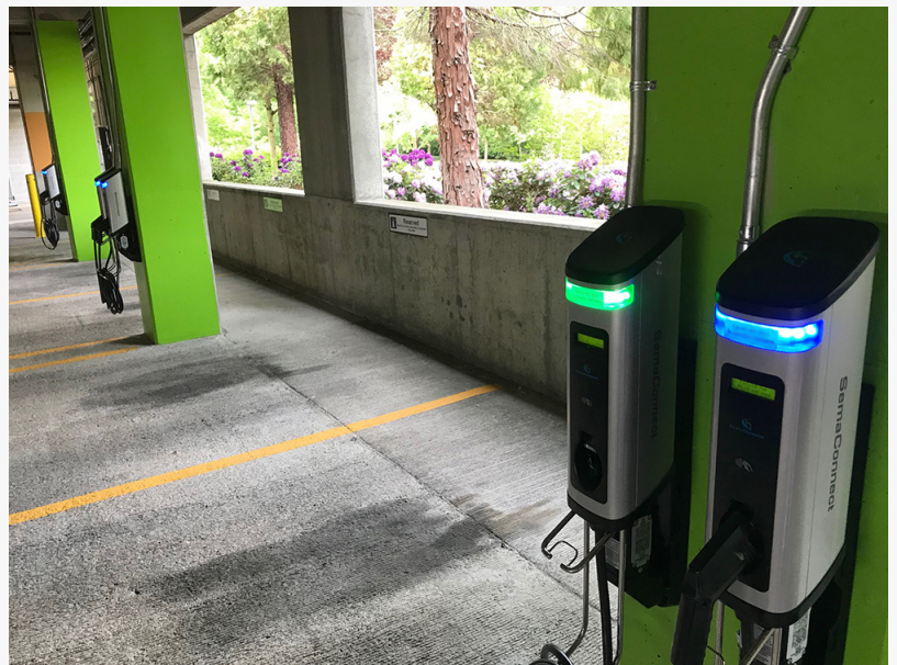
SemaConnect smart networked EV charging stations
