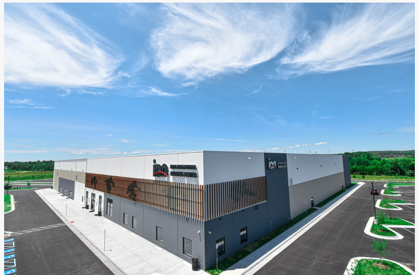
ION is located in Compass Creek in Leesburg, Virginia.
