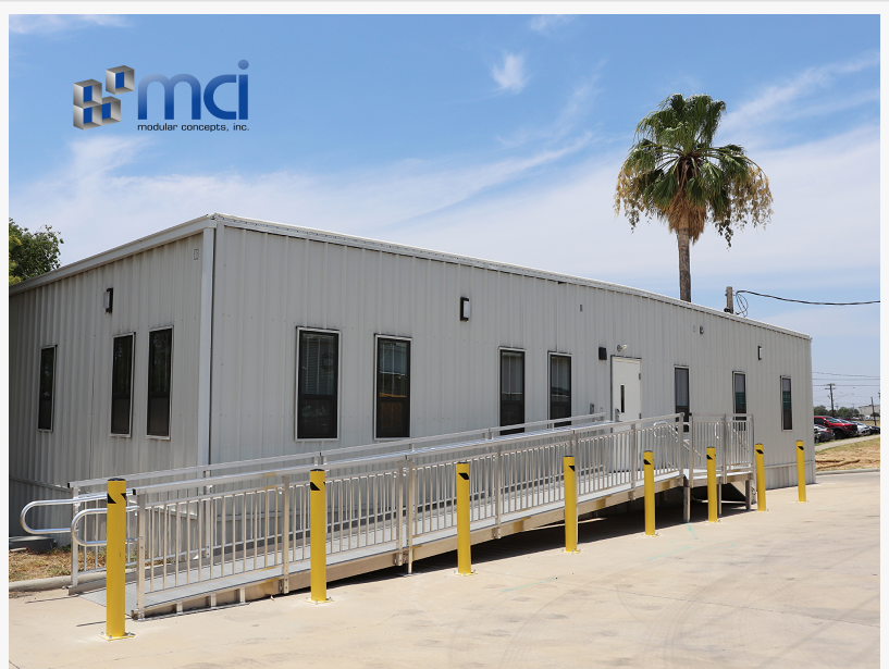
Exterior View of DHS-CBP Laredo Modular Administration Building.
