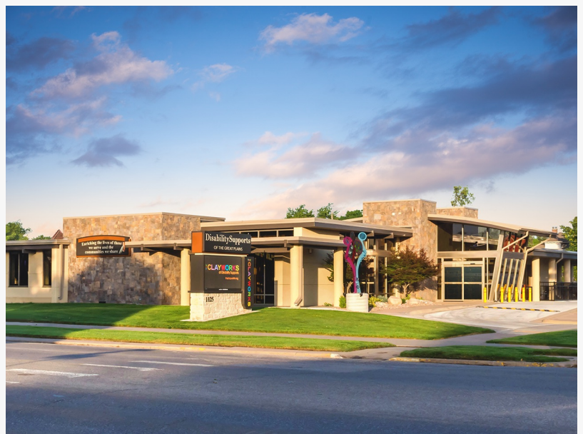
19,000 square feet commercial building completely rebuilt and remodeled for use by people with disabilities and the community.
