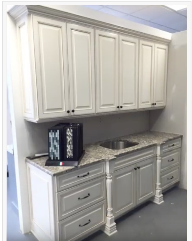
Installation of Custom Cabinets
