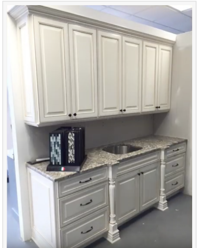
Installation of Custom Cabinets
