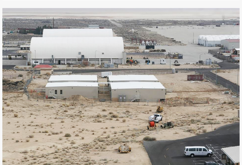
Modular Facilities at Edwards Air Force Base
