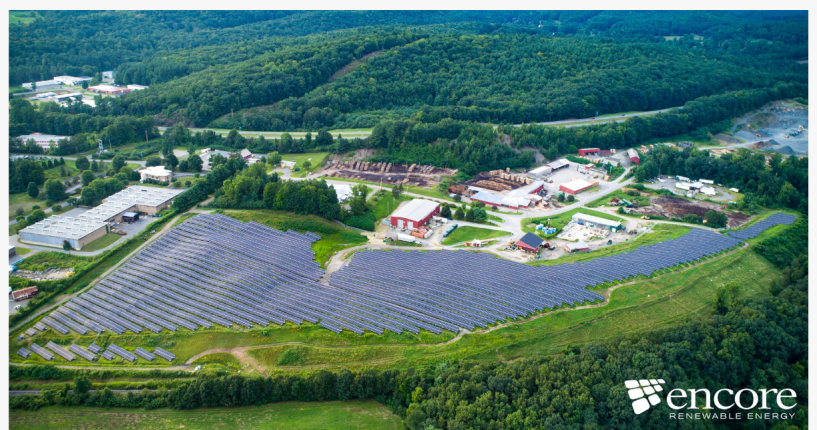
5.7MW array on the closed capped Brattleboro, Vermont landfill
