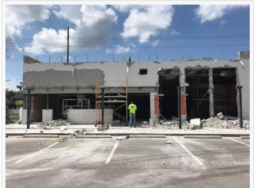
Dynamite Demolition Service Inc. Doing Concrete Demolition
