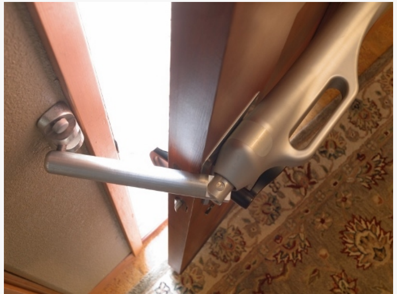
What a "security" chain is supposed to do - but doesn't.
