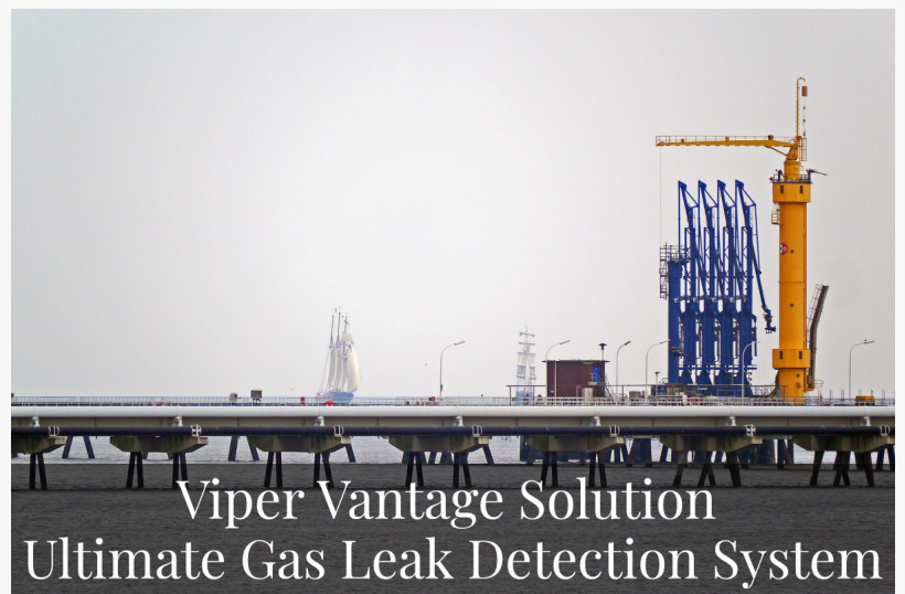
Viper Vantage - Ultimate Gas Leak Detection System - Production Facilities Inspection.
