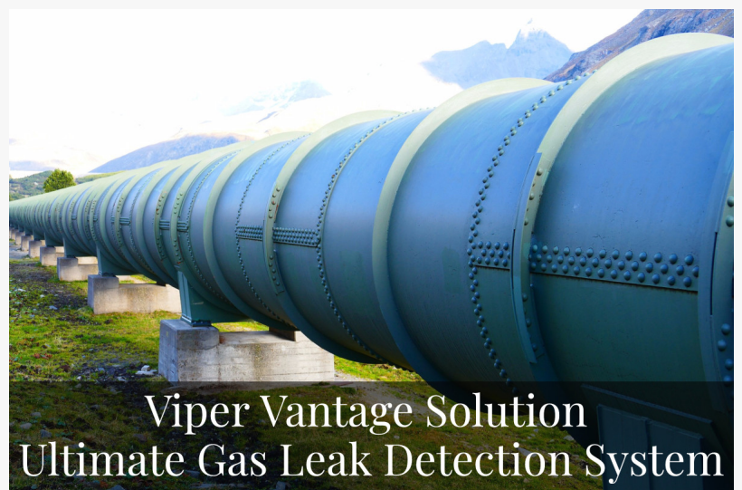
Viper Vantage - Ultimate Gas Leak Detection System - Extended Pipeline inspection
