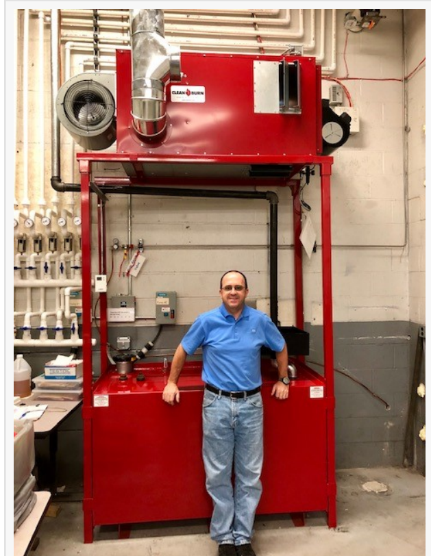
TestOil's Lucian Szokai with Waste Oil Furnace
