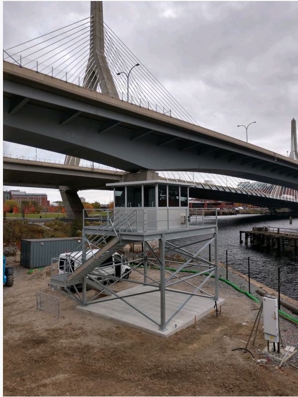
Boston's North Station Modular Building
