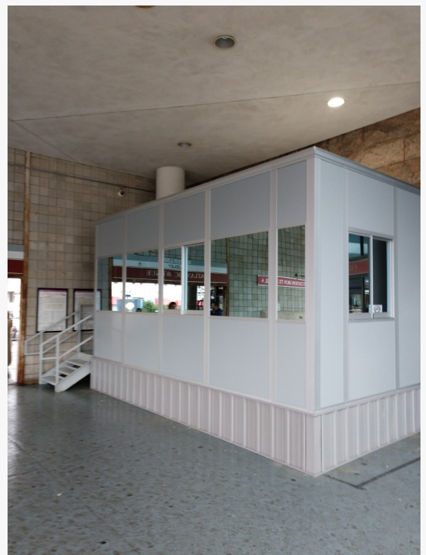
Boston's South Station Prefab construction
