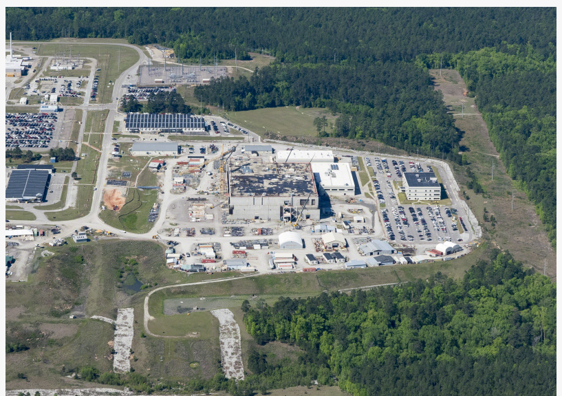
Abandoned plutonium fuel (MOX) building at Savannah River Site, courtesy High Flyer to SRS Watch
