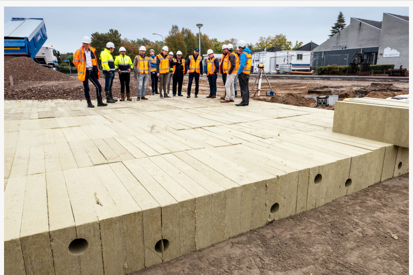
Urban renovation in the Netherlands: Rockflow is helping the Zonnemaat neighborhood prevent flooding from heavy rain.
