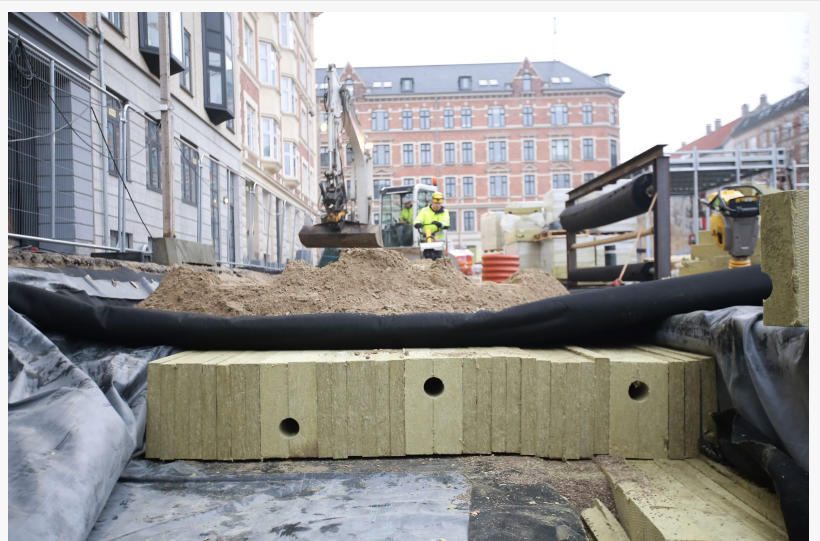
Rockflow is installed underneath Langeland Plads, a newly renovated public square in Frederiksberg, Denmark
