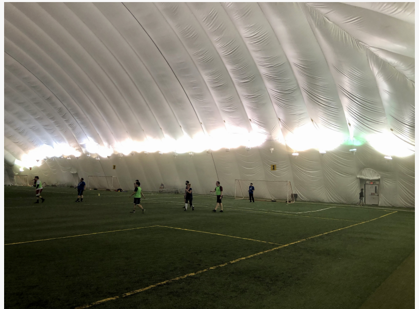
Sports Underdome Existing MH Lighting
