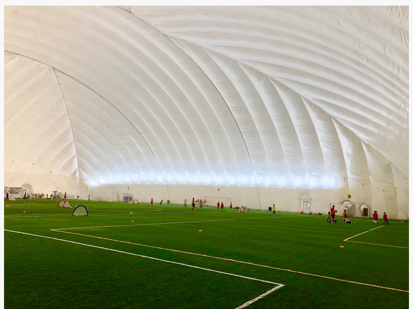
Sports Underdome New Eclipse Lighting
