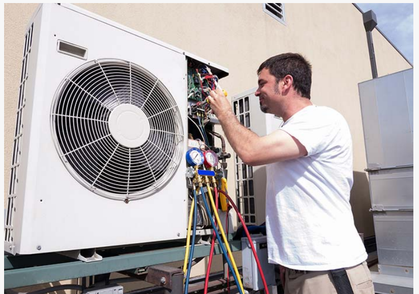
AC Repair in Houston TX
