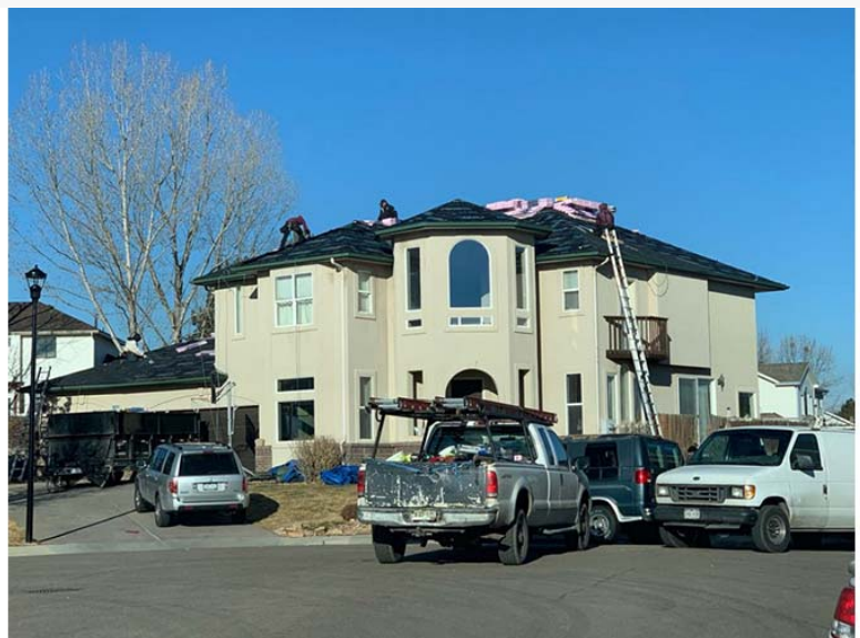
roof repair project in Fort Collins, CO
