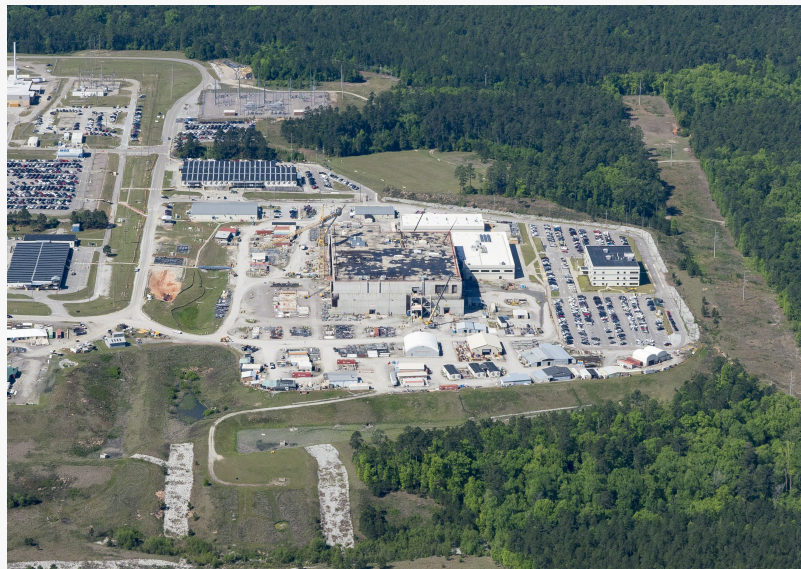
Abandoned plutonium fuel (MOX) building at Savannah River Site, Not Suited to become a Plutonium Bomb Plant (PBP), courtesy High Flyer - ©2019SCHighFlyer - to SRS Watch
