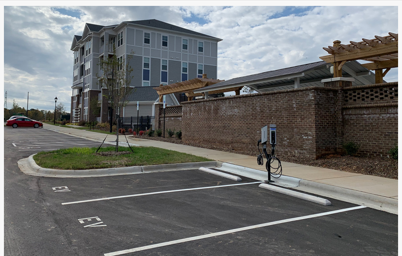
The new SemaConnect EV charging stations at Riverbend Apartments make life easier for residents with electric vehicles
