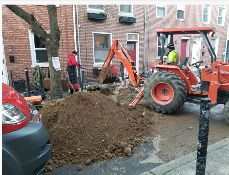
repairing broken pipes
