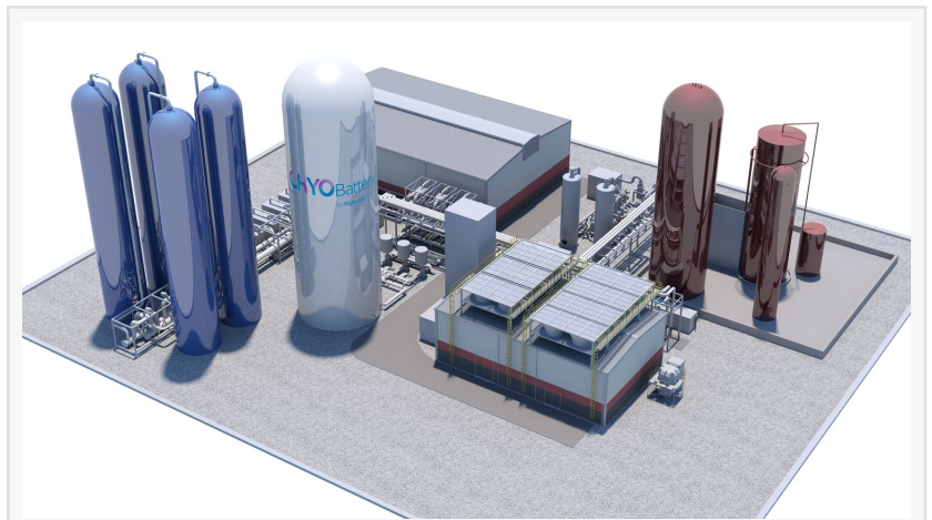
This is a standard configuration for a Highview Power long duration, liquid air energy storage system.
