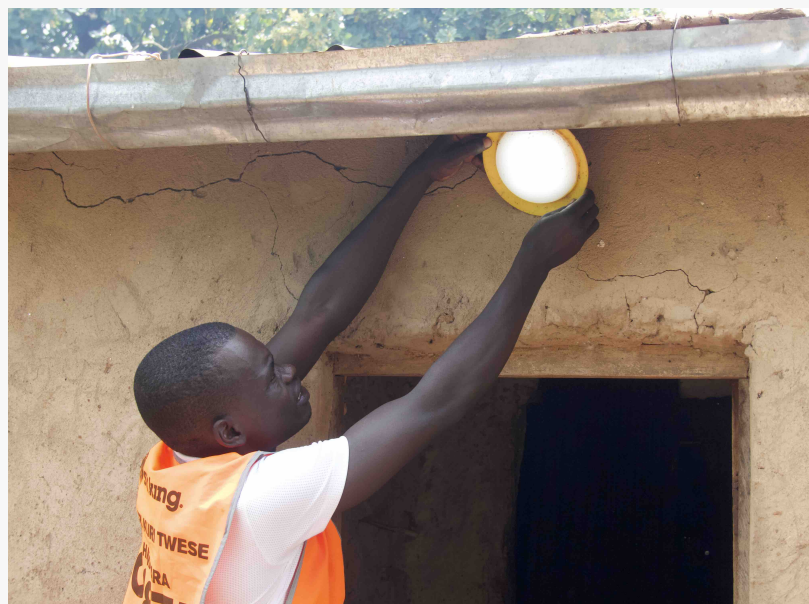
Home system installation
