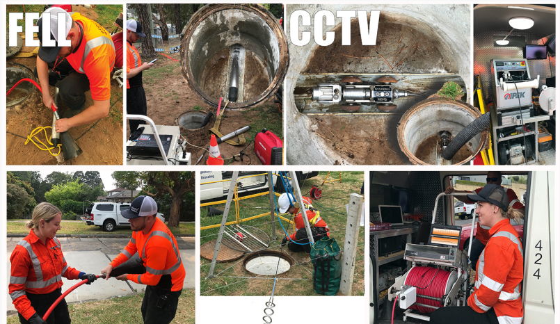
Electro Scan field crew performing FELL with comparisons to CCTV.
