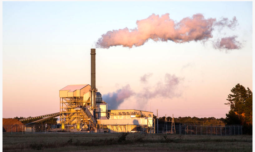
Woody Biomass Plant - Lufkin, TX
