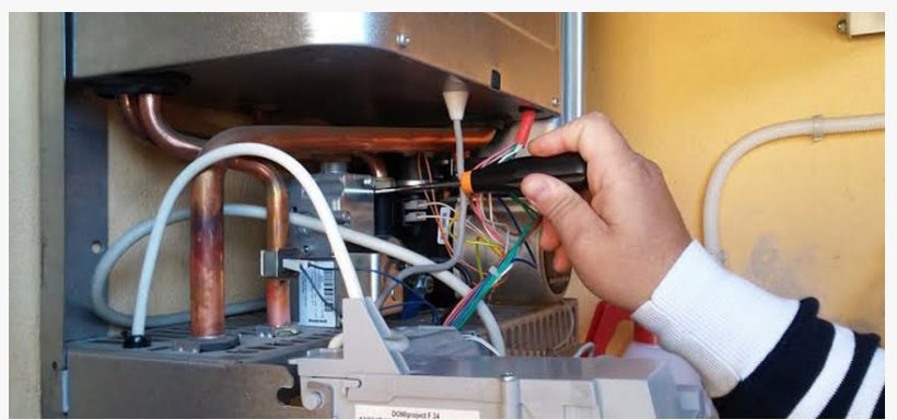
Furnace Repair in Frisco TX
