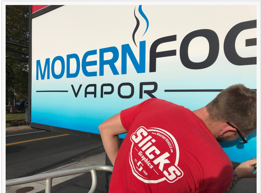
Slicks Graphics installing a custom illuminated sign.
