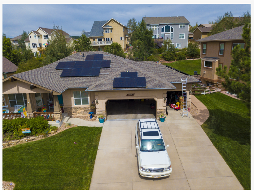
Sunfinity designed and installed this solar system for a Colorado homeowner.
