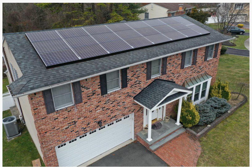
Another drone image of an installation that was completed by the SUNation team!
