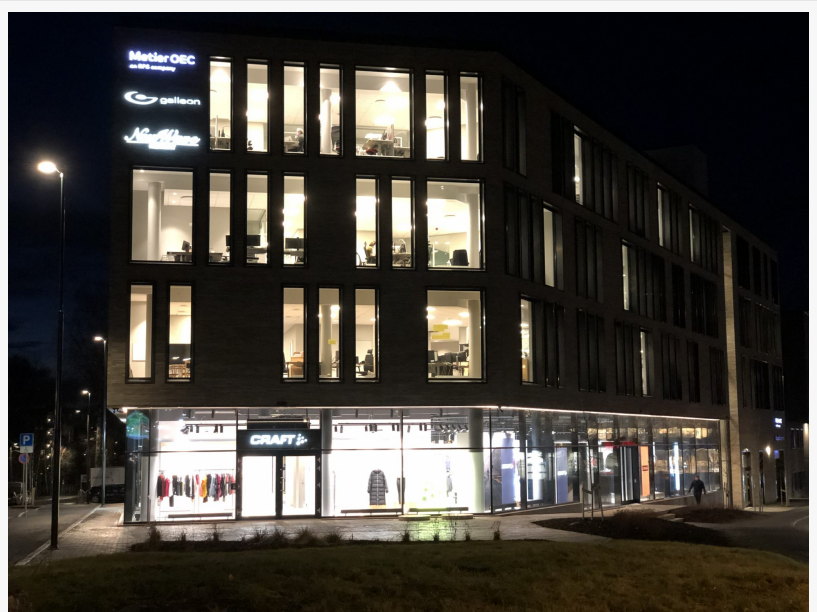
Galleon Office Building Oslo
