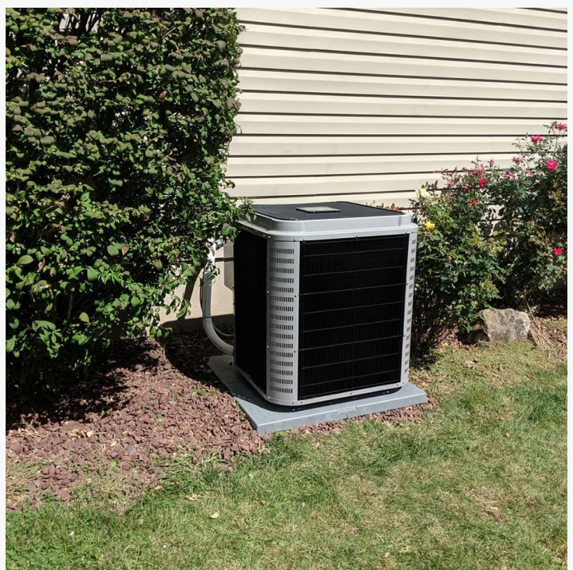
Nice and clean area around this AC compressor unit!
