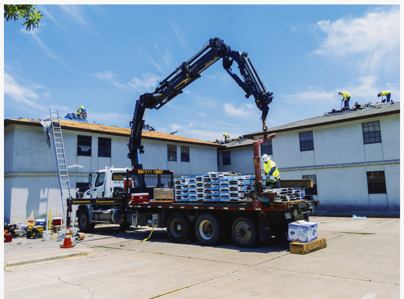
McAllen Valley Roofing Co. roofing contractors repairing a damaged apartment complex.
