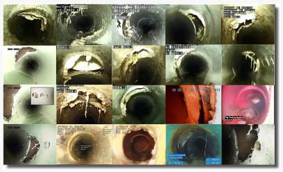
Example defective customer reconnections, after CIPP installation and lateral reinstatement.
