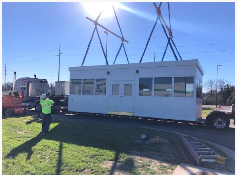
Modular Security Building Delivery Irving GA
