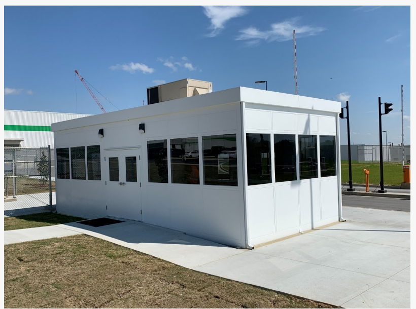
Prefab Security Building Installed Irving Tissue Company
