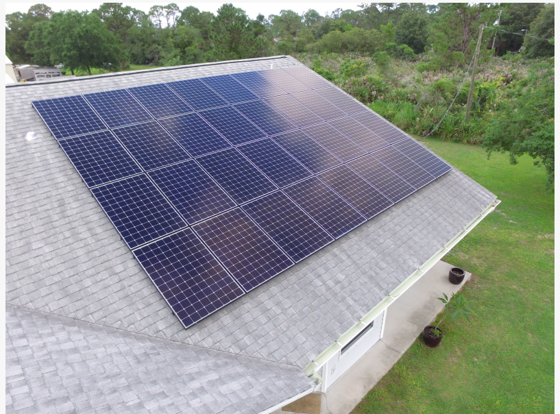
SunPower Rooftop Solar Panels
