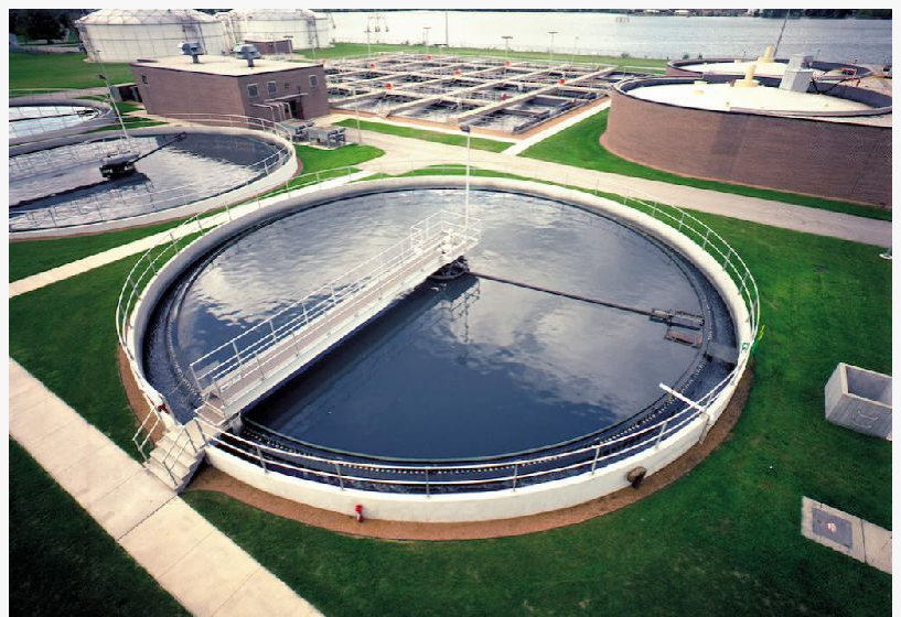
Wastewater Treatment Services
